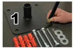
Place base plate in desired anchoring location
