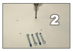
• Using a 1/2" masonry bit, drill 5" in depth
