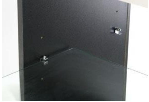
Step 11: Flip unit right side up. Insert shelf pegs at desired heights. (You may need a rubber mallet – the pegs are a tight fit).
